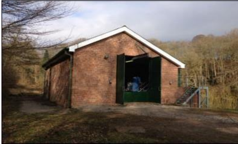
Figure 5: River Eden intake – showing flood protection door
