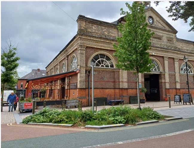
Figure 21: SuDS within Altrincham
