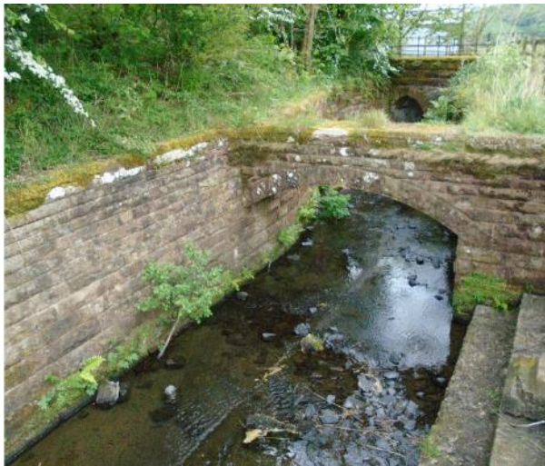
Figure 3.14 : Reinforced channel (facing downstream)
