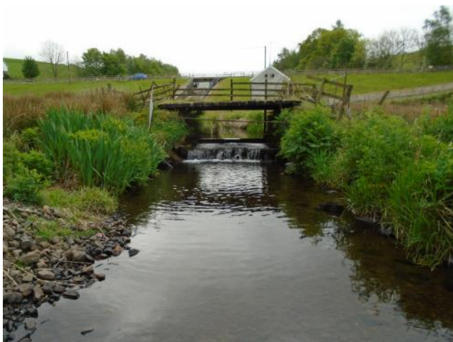
Figure 3.17 : Immediately downstream of Chapelhouse Reservoir (facing upstream)
