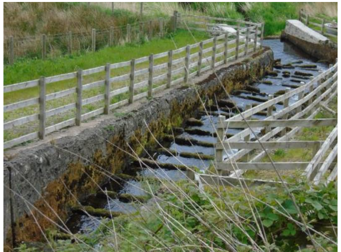
Figure 3.15 : Stepped fish pass on dam face (facing downstream)
