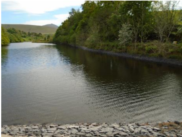
Figure 3.16 : Chapelhouse Reservoir (facing upstream)
