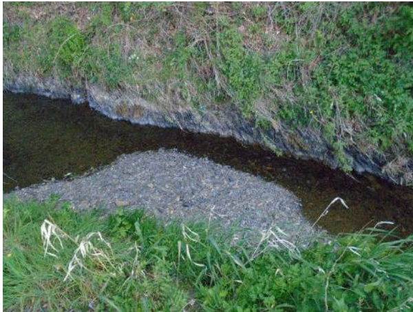
Figure 3.12 : Bypass channel with small deposit (facing the left bank)
