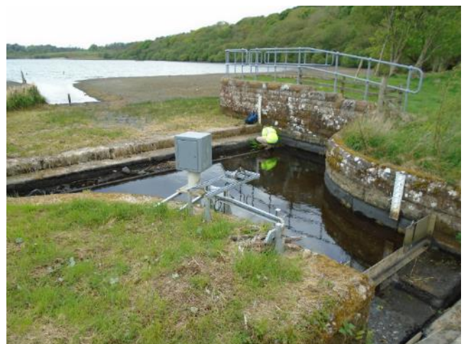
Figure 3.29 : Weir infrastructure at downstream extent of Over Water (facing upstream)
