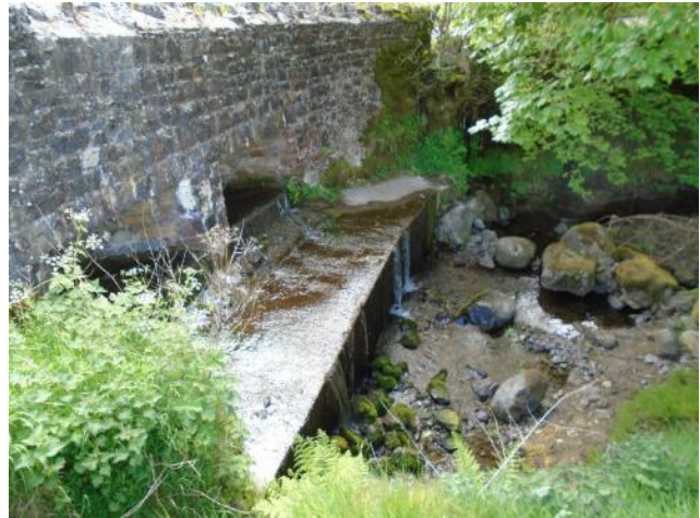
Figure 3.23 : Weir downstream of local access road (facing left bank)
