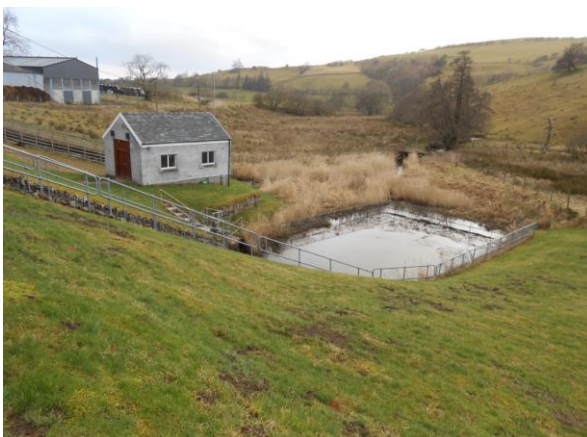
Figure 4-3: Chapelhouse reservoir downstream slope
