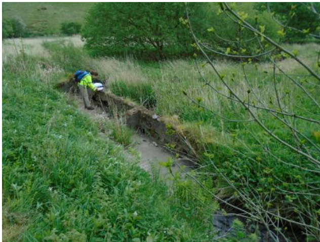
Figure 3.10 : Redundant sluice structure (facing downstream)
