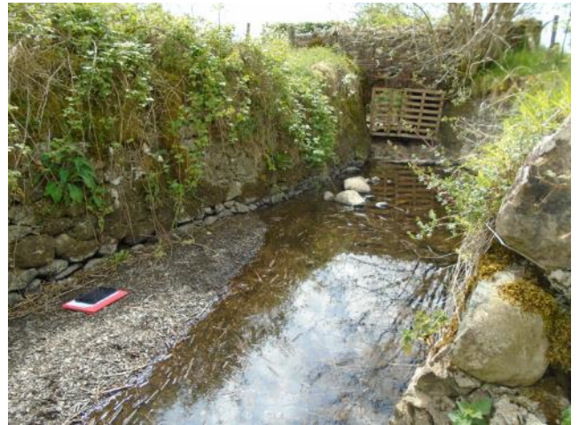
Figure 3.33 : Over Water channel culvert under access road (facing upstream)
