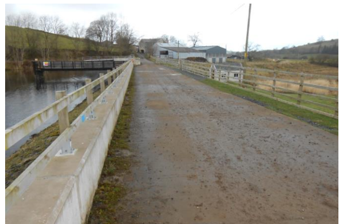
Figure 4-4: Chapelhouse reservoir embankment crest
