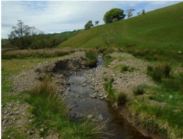
Figure 3.26 : Material on channel bank tops (facing downstream)
