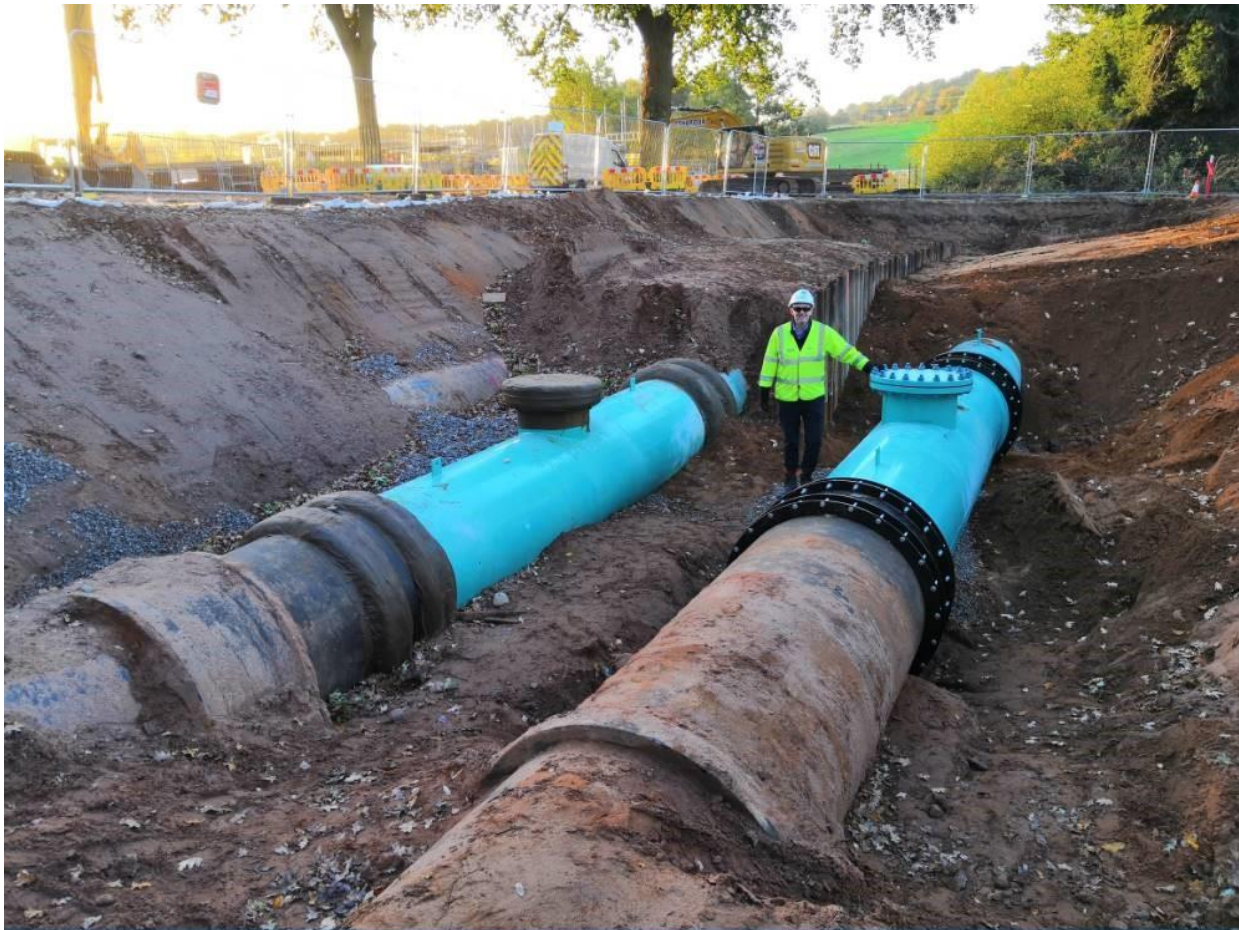
Figure 2. Photograph demonstrating the scale of the Vyrnwy Aqueduct. This shows two lines of the potable section during recent diversion works in Cheshire.
