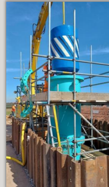
A 'pig' being lowered into the aqueduct
