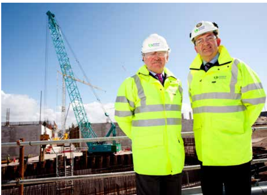
Pictured: Dr John McAdam (far left) and Steve Mogford on a board visit to Liverpool wastewater treatment works. The site is undergoing a £200 million expansion to handle up to 11,000 litres of wastewater every second, serving a population of more than 600,000 people and industry. The project is set to create 350 jobs and is scheduled for completion in 2016.
