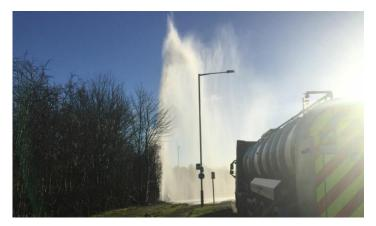
Figure 9: Burst on a 10" polyvinyl chloride main in Chorley, 2018
