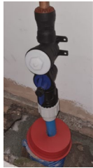
Meter housing unit incorporating all the required fittings
