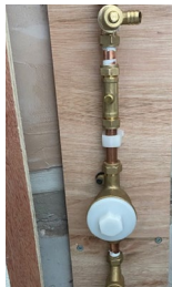
Separate meter housing together with blanking plug, BS1010 stop tap, in-line double check valve and drain off
