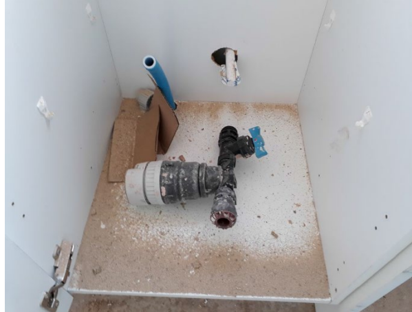
Internal meter install poor practice
