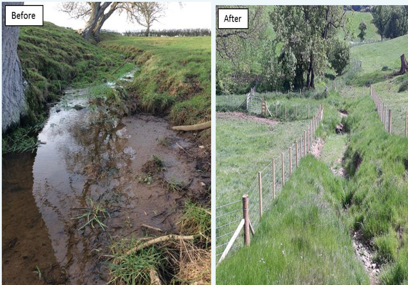
Figure 6: Fencing and silt pond reduces bankside erosion and slows the flow during heavy rain
