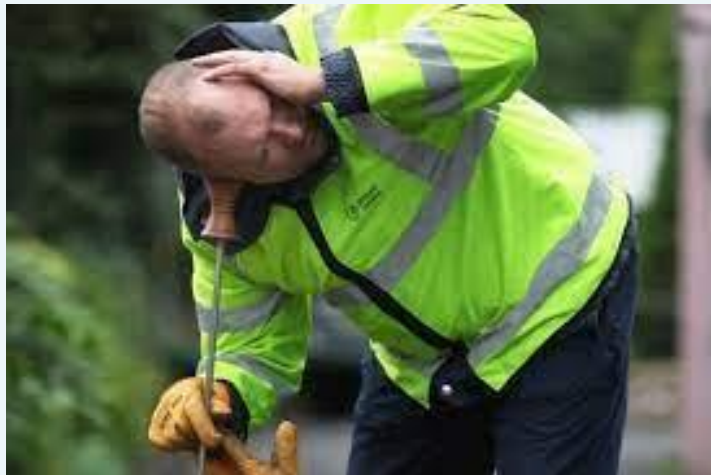
Figure 3: Leakage technician using conventional leak detection methods
