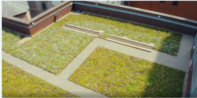
Figure 7: The retrofit blue/green roof on Bruntwood Bloc in Manchester
