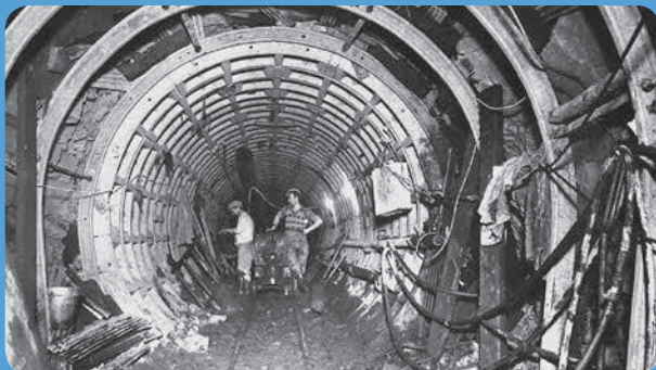
PHOTOGRAPH: Construction of the Haweswater aqueduct started in 1933 and took more than 20 years to complete.
