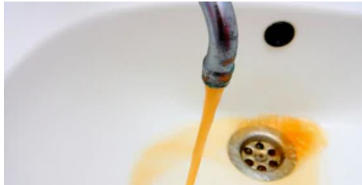
Discolouration of water
