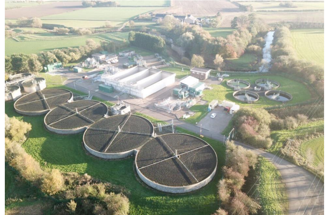
Garstang Sewage Treatment Works
